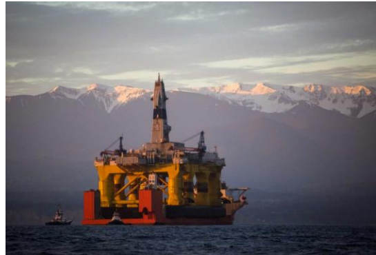
Shell's Kulluk drilling rig grounded near Kodiak, AK. Photo Credit: U.S. Coast Guard
